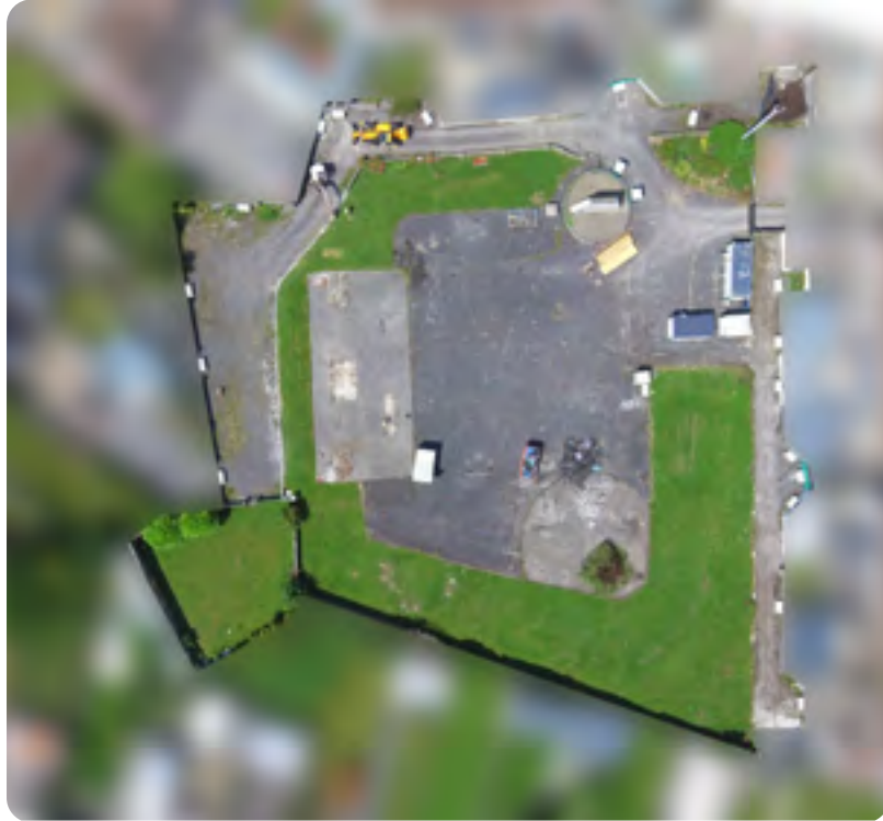
Aerial image of site before commencement of excavation in July 2025
