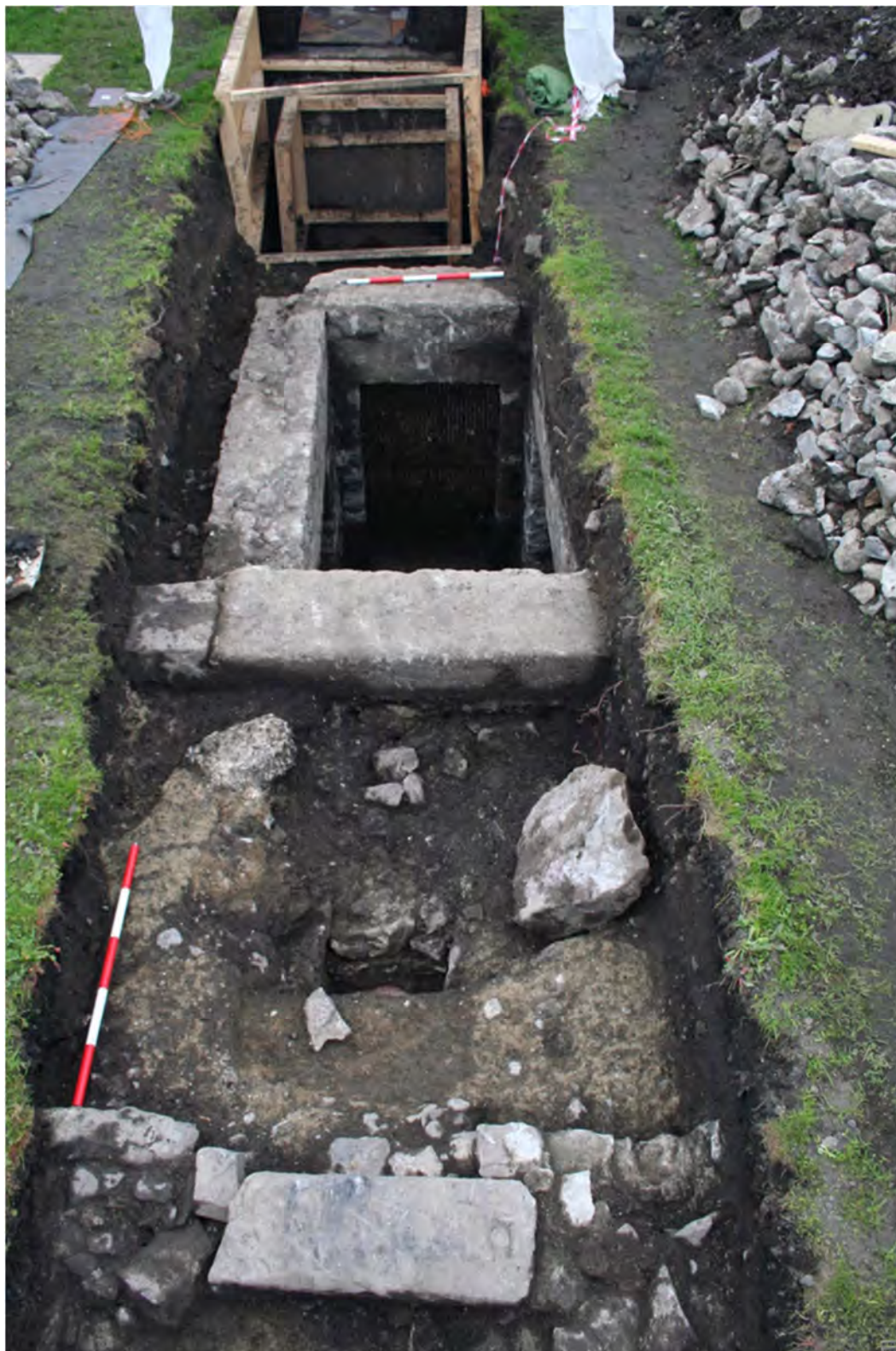
Plate 2.3: Culvert and tank associated (Feature 2/C.8)
