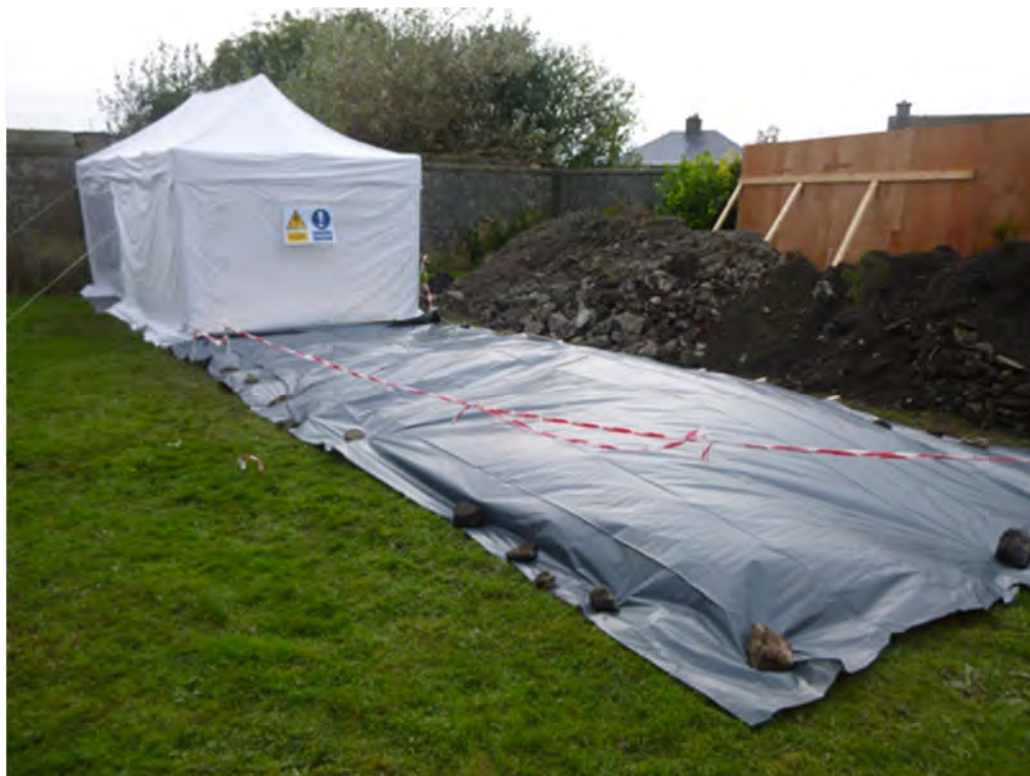
Plate 1.4: Securing excavations on site
