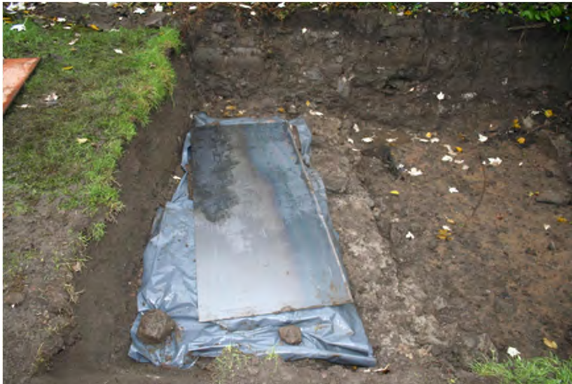
Plate 6.1: Sealing of chambers prior to backfilling site
