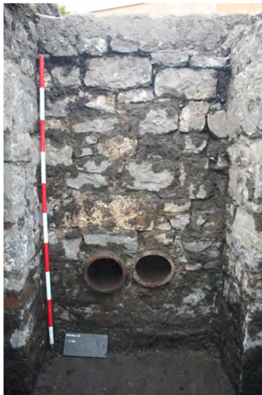
Plate 2.7: North wall of tank with inlet pipes
