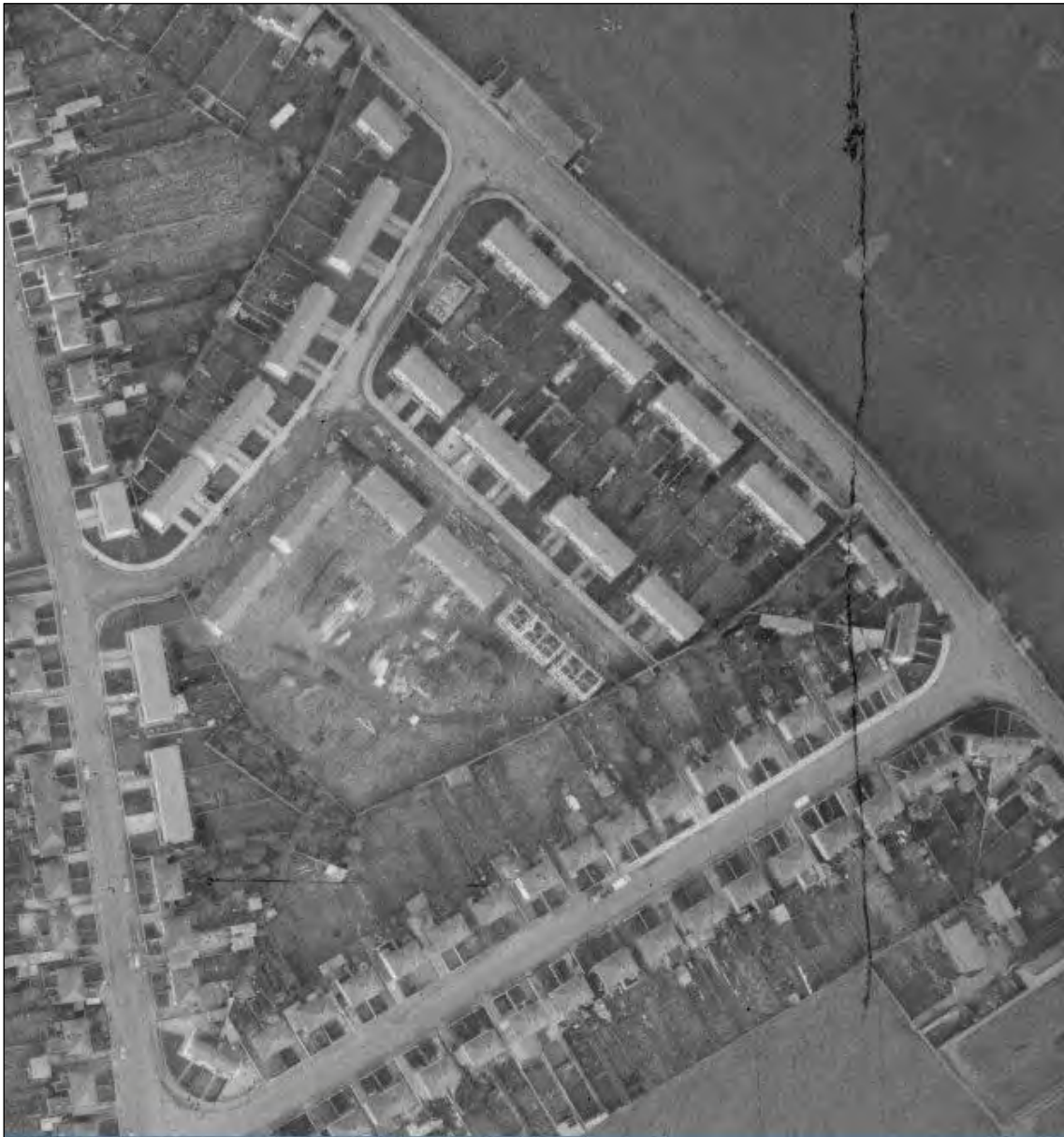
Figure 11: Aerial photograph of the site in the final stages of redevelopment in 1977 reproduced at kettleontherange.com
