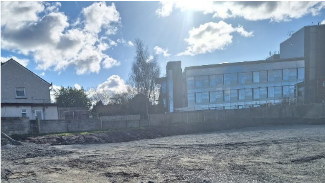
Figure 4: Example of berm excavation.
