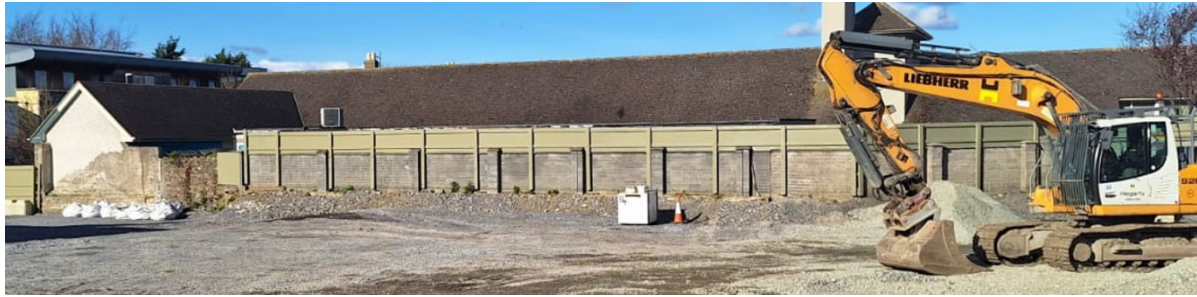
Figure 5: Example of privacy hoarding to boundary walls.
