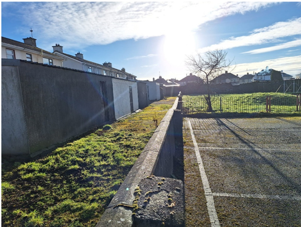
Image 3: Pedestrian access to rear gardens of Dublin Road estate
