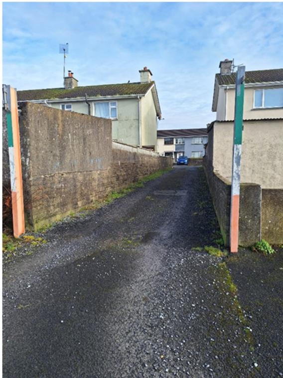
Image 1: Entrance from interior side of Dublin Road Estate (approx. width 3.3m)
