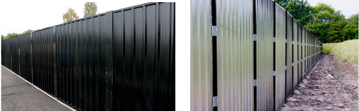
Figure 7: Example of sheet metal hoarding (front and rear)
